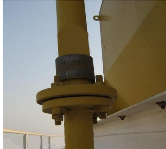
Fig. 55: Incompatible Ring Main Branch Pipe and Foam Pourer Flange Sizes
