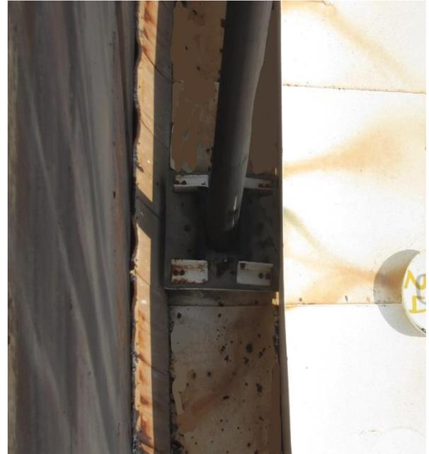
**Fig. 11:** Foam Blockage by Guide Pole Due to Poor Design of Foam Dam
