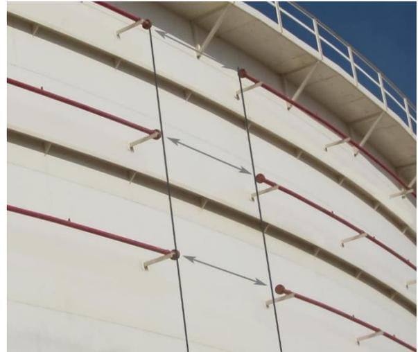
**Fig. 30:** Dry Strip Due to Inadequate Nozzle Separation Distance
