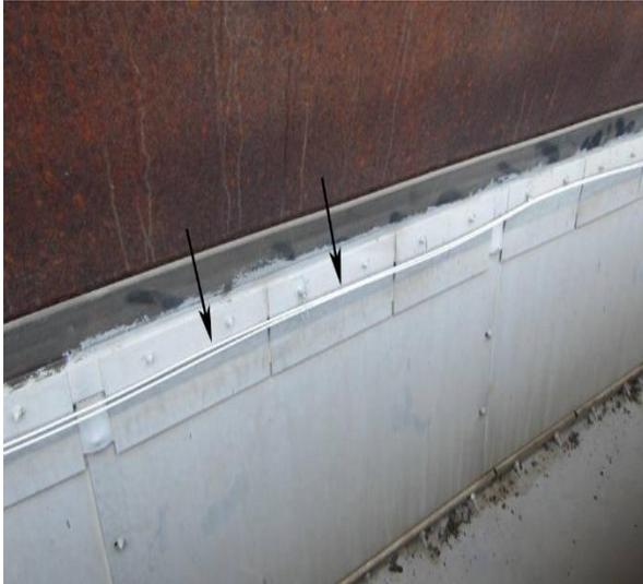
**Fig. 57:** Linear Heat Detector
