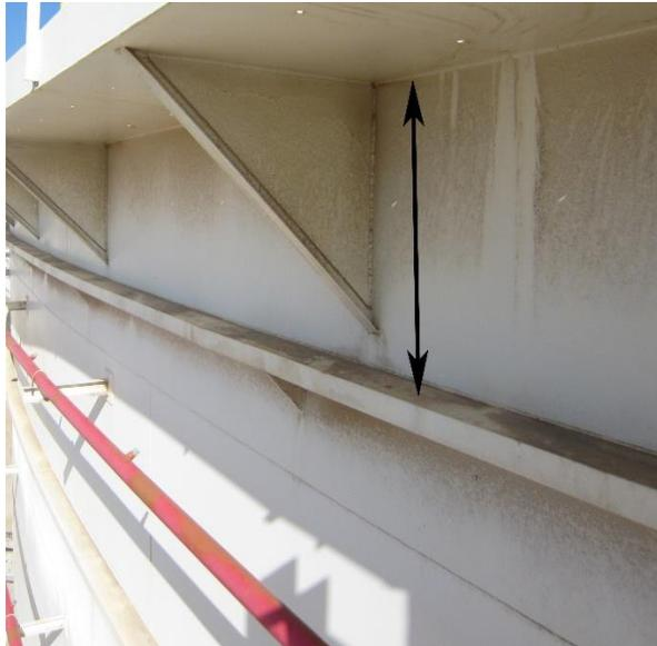
**Fig. 28:** Providing No Cooling Ring above Wind girder
