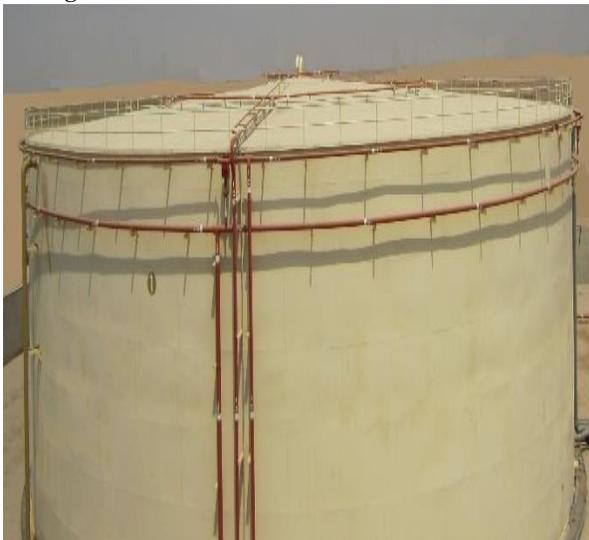
**Fig 33:** Cooling System for Shell and Roof of a Fixed Roof Tank
