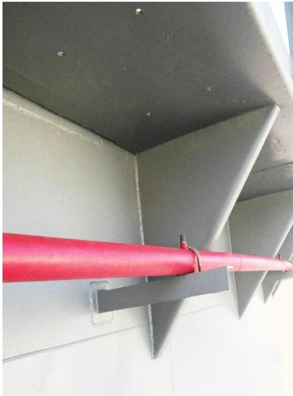
**Fig. 13:** Water Curtain Blockage by Triangular Support Members
