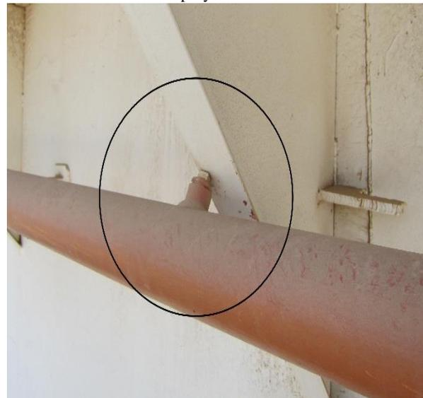
**Fig. 27:** Blockage of Outlets by Tank Appurtenances
