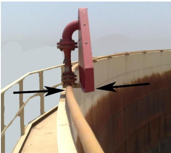
**Fig. 49:** Foam Pourer Sticking inside the Tank
