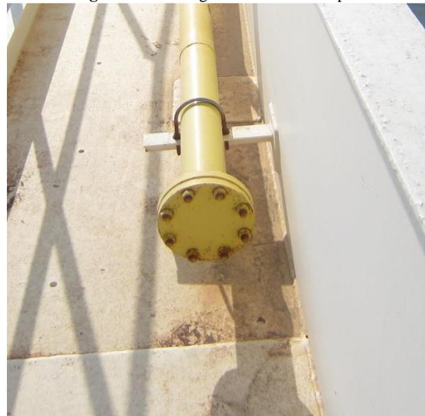
**Fig. 60:** Foam Ring Main with Flanged End
