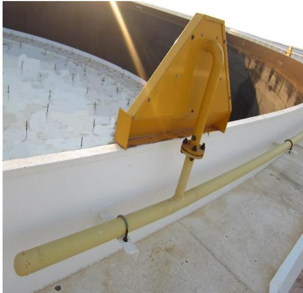
Fig. 53: Foam Solution Ring Main Above Walkway
