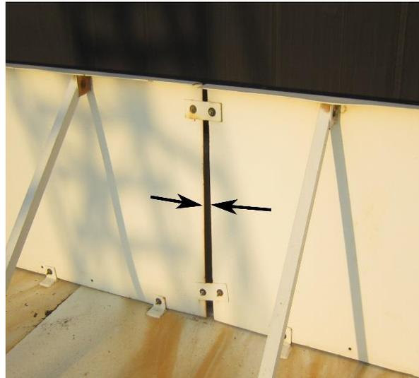
**Fig. 4:** Foam Dam Fastening Using Nuts and Bolts
