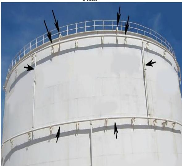
**Fig 34:** Connected Roof and Shell Water Spray Cooling System
