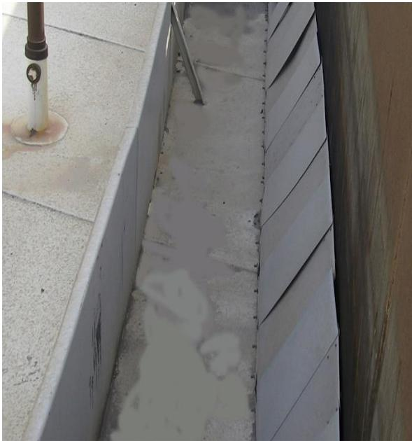
**Fig. 10:** Inappropriate Foam Dam Width
