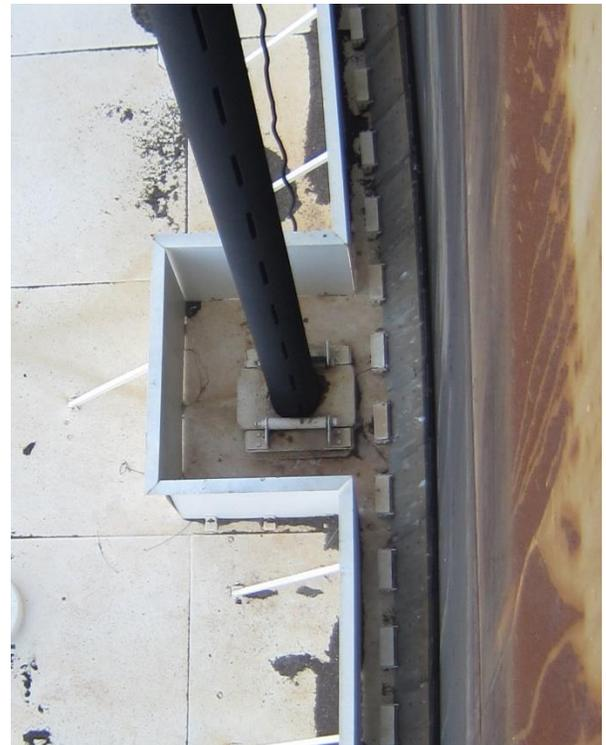
**Fig. 12:** Good Design of Foam Dam around Guide Pole
