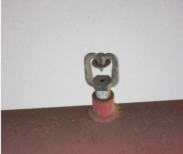
**Fig. 23:** Inappropriate Spray Nozzle - Full Cone Medium Velocity Nozzle
