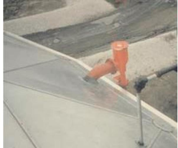
**Fig. 50:** Installation of Foam Pourer on the Roof of Fixed Roof Tanks
