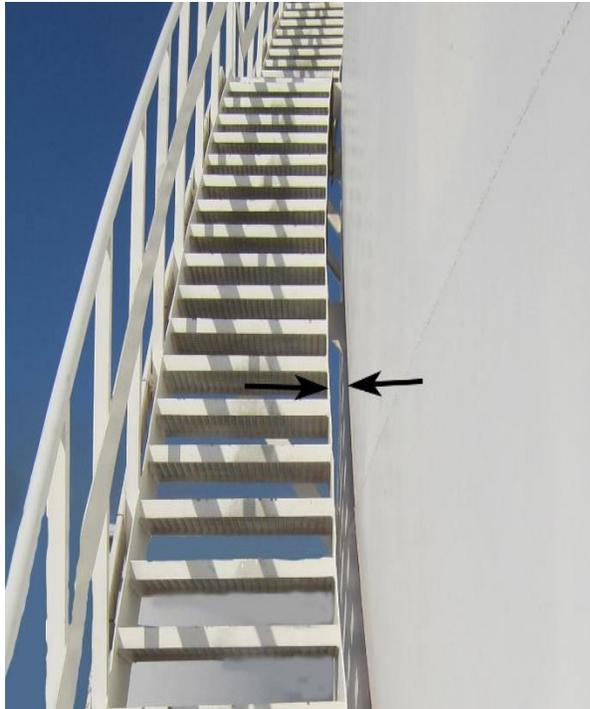
**Fig. 20:** Spiral Stairway Separated from Tank Shell
