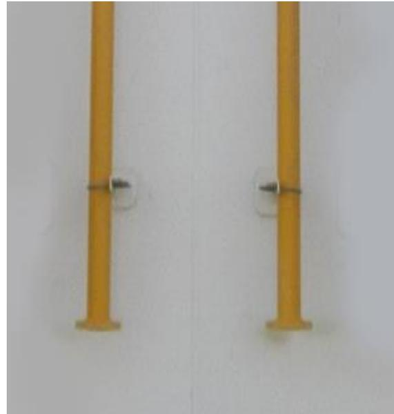
Fig. 42: Foam System with No Fire Department Connections
