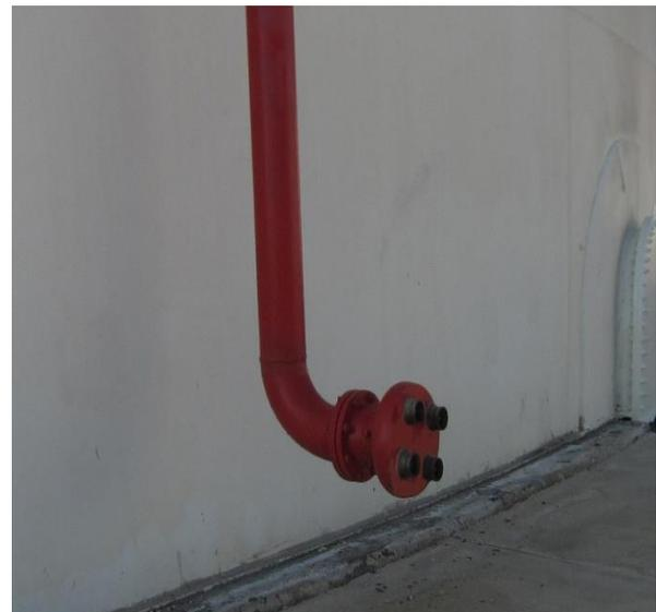
**Fig. 21:** Piping Terminated at Tank Bottom
