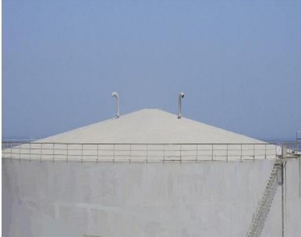
**Fig. 32:** Fixed Roof Tank with No Roof Protection
