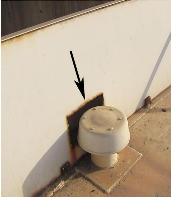
Fig. 5: Detrimental Foam Dam Modifications
