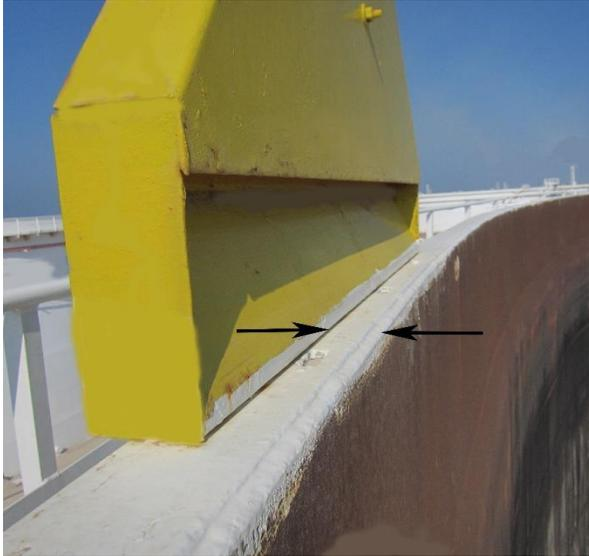
**Fig. 47:** Foam Pourer Positioned with Indentation from Inner Tank Wall
