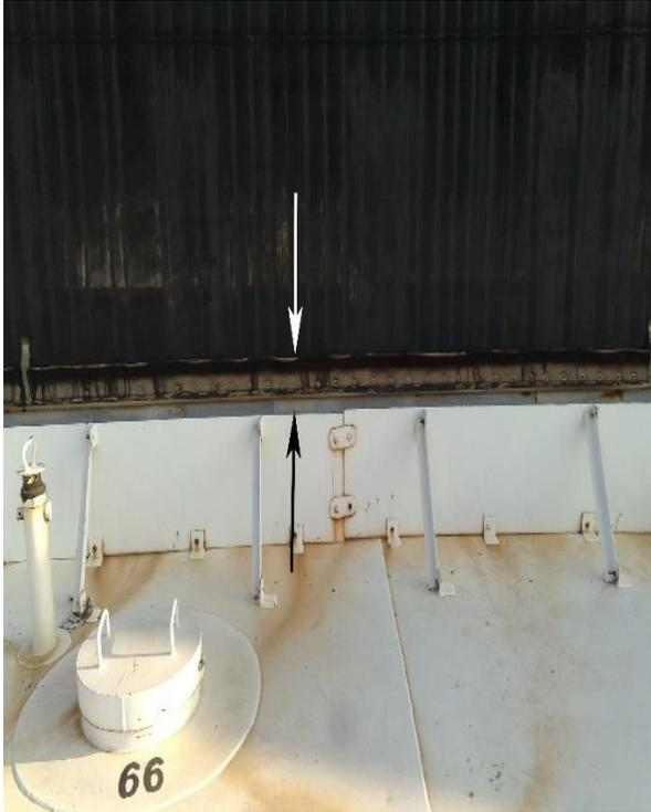
**Fig. 9:** Inappropriate Foam Dam Height
