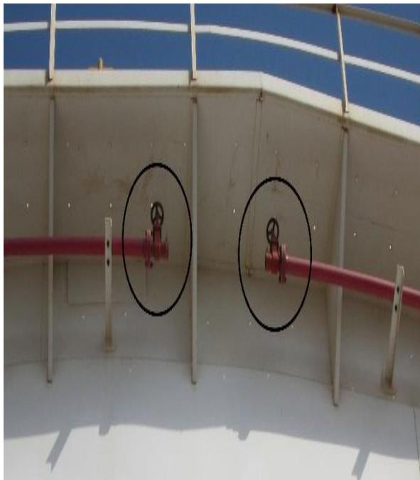
**Fig. 38:** Ring Main with a Valve at the End
