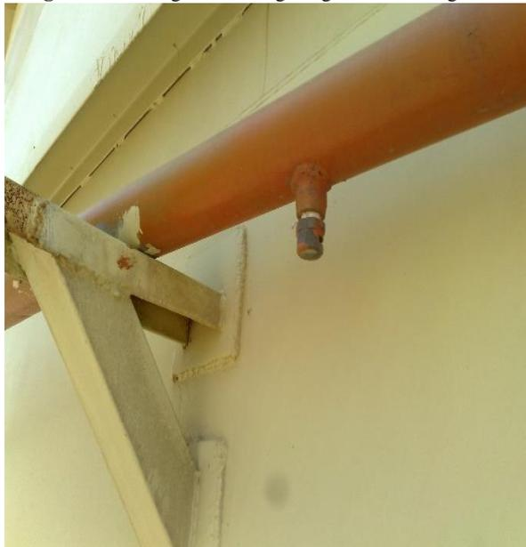
**Fig. 29:** Water Spray Nozzles Installed in 6 O'clock Position of Ring Main
