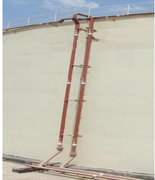
**Fig. 35:** Separated Roof and Shell Water Spray Cooling System
