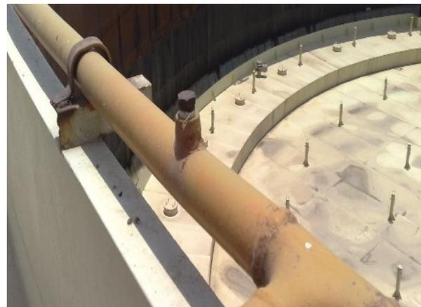
Fig. 56: Tap for Pressure Gauge
