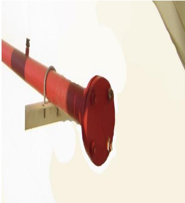
**Fig. 37:** Ring Main with Flanged End
