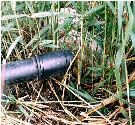
**Fig.2:** Septic effluent pipe entering to polishing natural wetland in the research site
